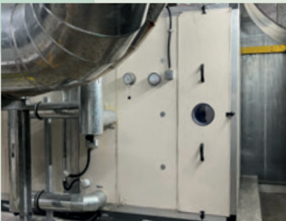
Selected AHU in Terminal 3 with the EC FanGrid installed
