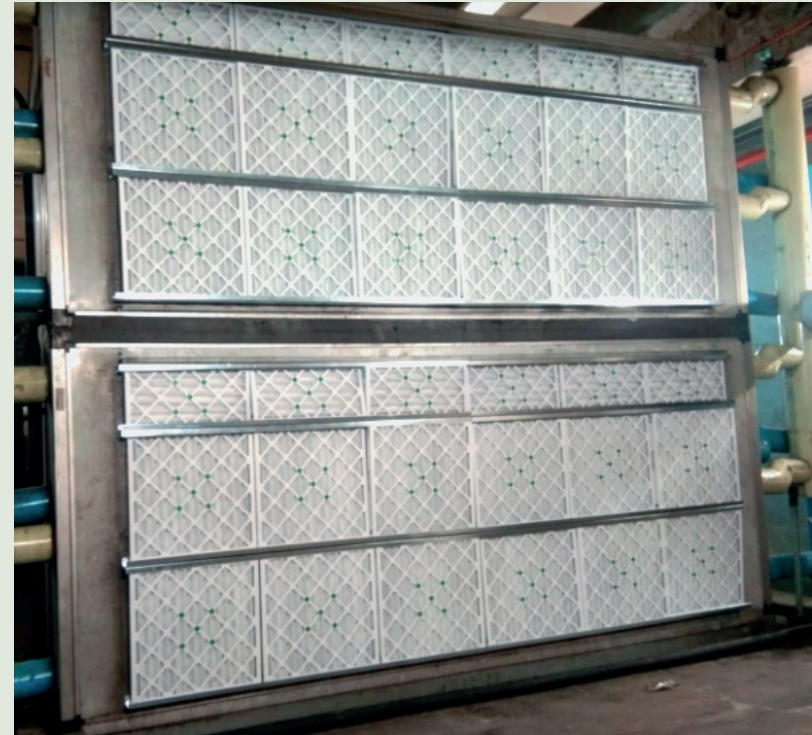
MERV 14 filters used in Terminal 2's Air Handling Station
